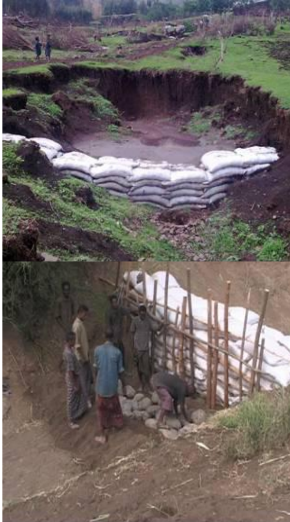
Sandbag check-dams constructed to treat medium sized gullies
