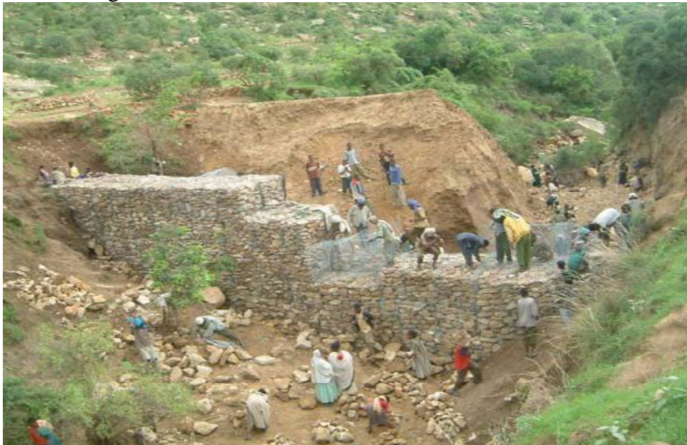
Gabion check-dam under construction
