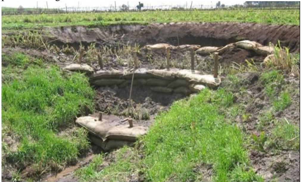
Gully head control with sand bags and other vegetative measures.
