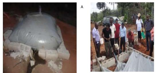
Fig. 4.1 (a) & (b): Construction of Flexible Tank Biogas Plant and the Plant with Full Gas Yield. Photo taken at Federal University of Technology Owerri).
