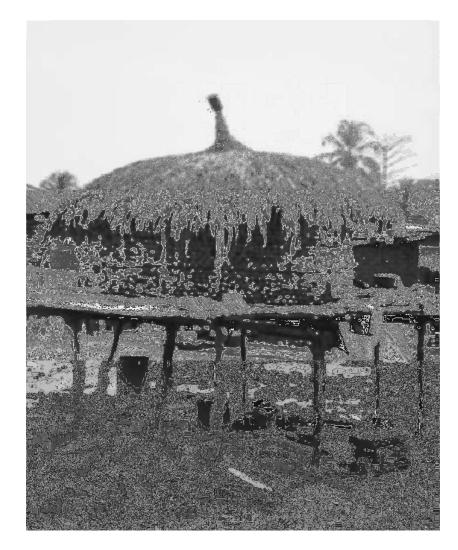
Fig. 5: Timber platform frame
