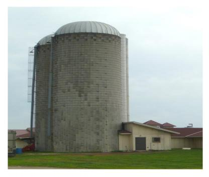
Figure 5. Concrete stave tower silos.
